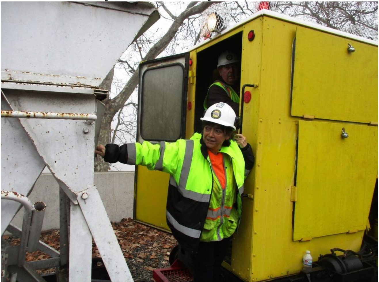
Pam relays signals from the brakeman for Harry in the tie-shear whose vision is obstructed by hopper cars
