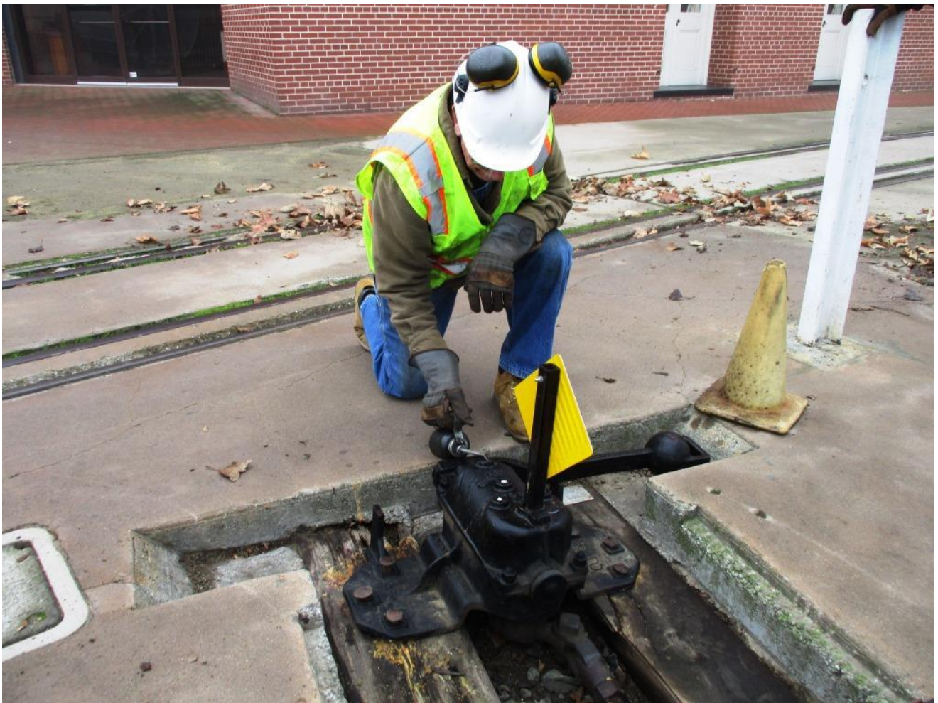
Clem oils the switch machine at Switch 1
