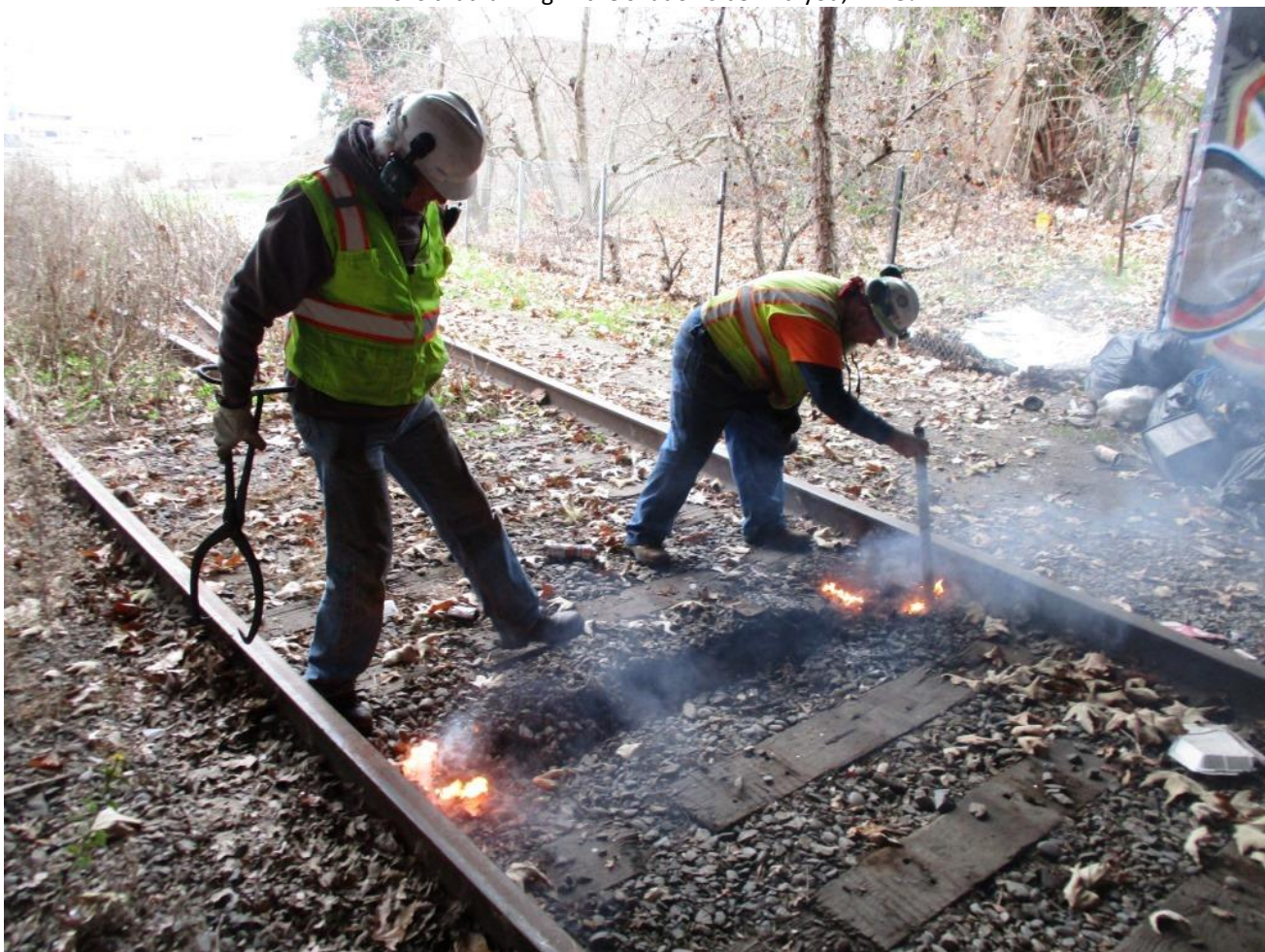
Steve and Mike F. find a fire in the tunnel at Setzer and work to smother the flames
