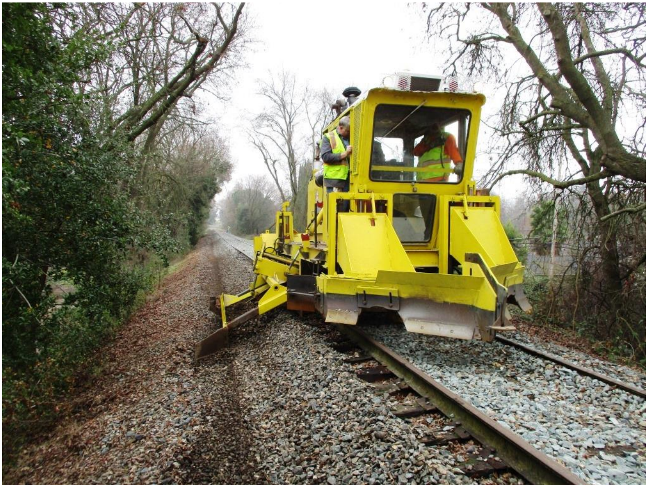
Chris C. in the ballast regulator uses the wing to pull rock up towards the track from the shoulder
