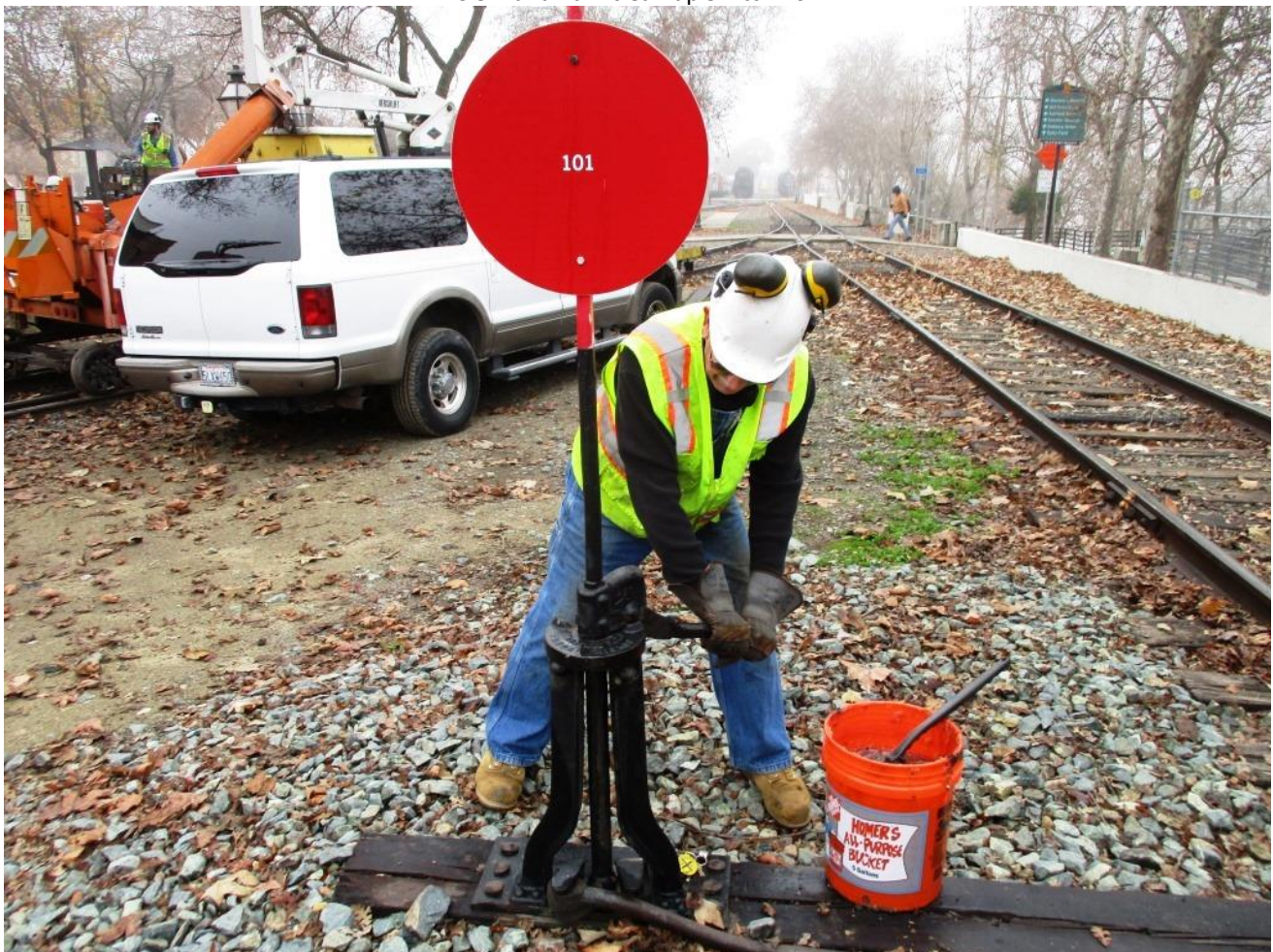
With the switch serviced and greased, Clem exercises the switch machine
