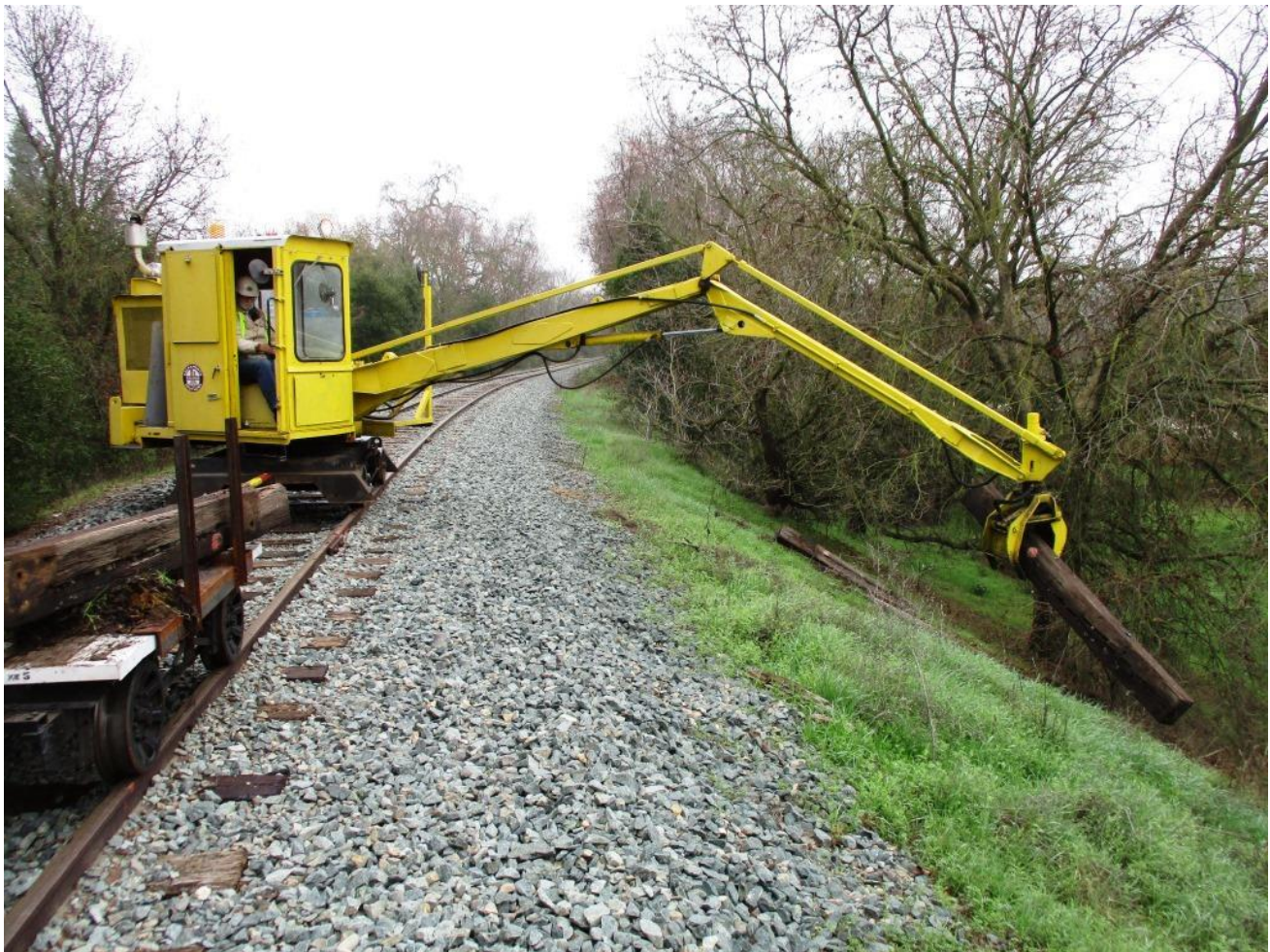
Alan in the tie-crane stretches out the boom to grab a dead-tie
