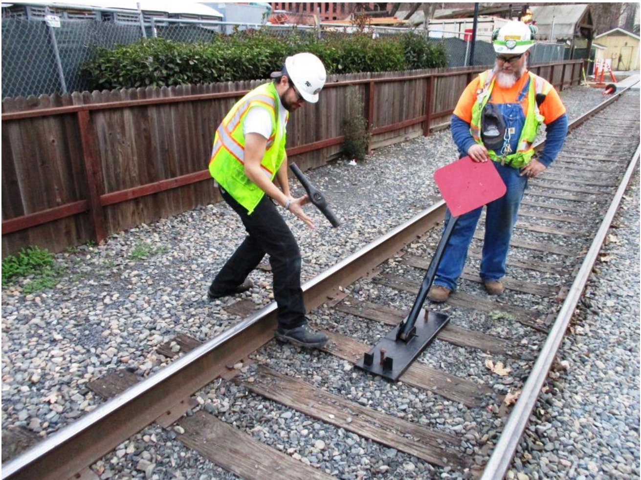
At Mile Post 3.0 in Old Sac., Mike F. holds the retractable red-flag as Kyle attempts to spike it to the tie
