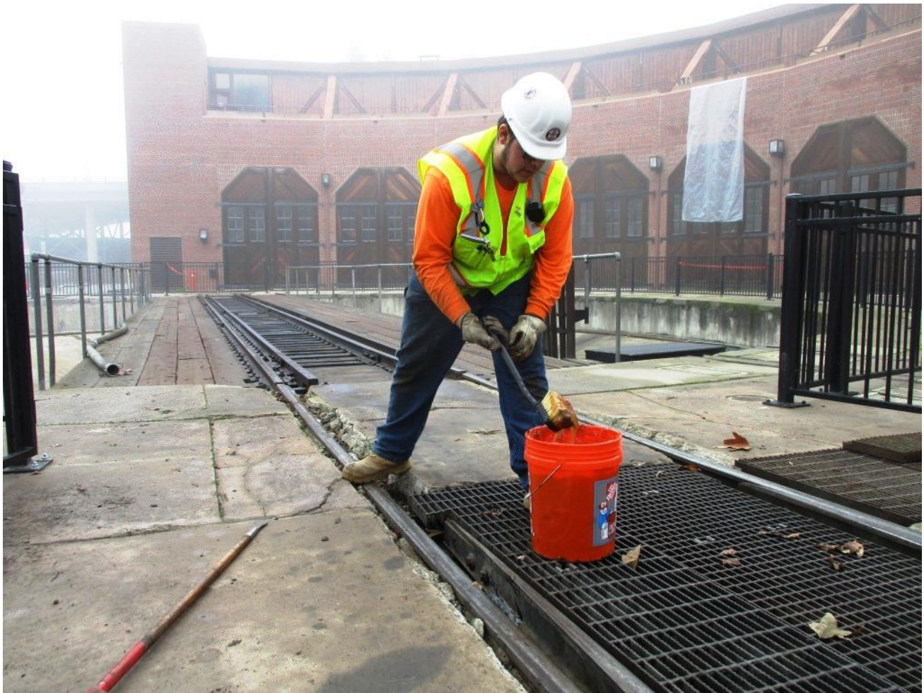
That magic moment has arrived: Chris H. greases the plates at Switch 1
