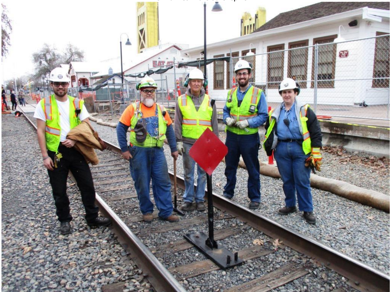
And, with that, Kyle, Mike F., Steve, Weston, and Heather declare another good job done!
