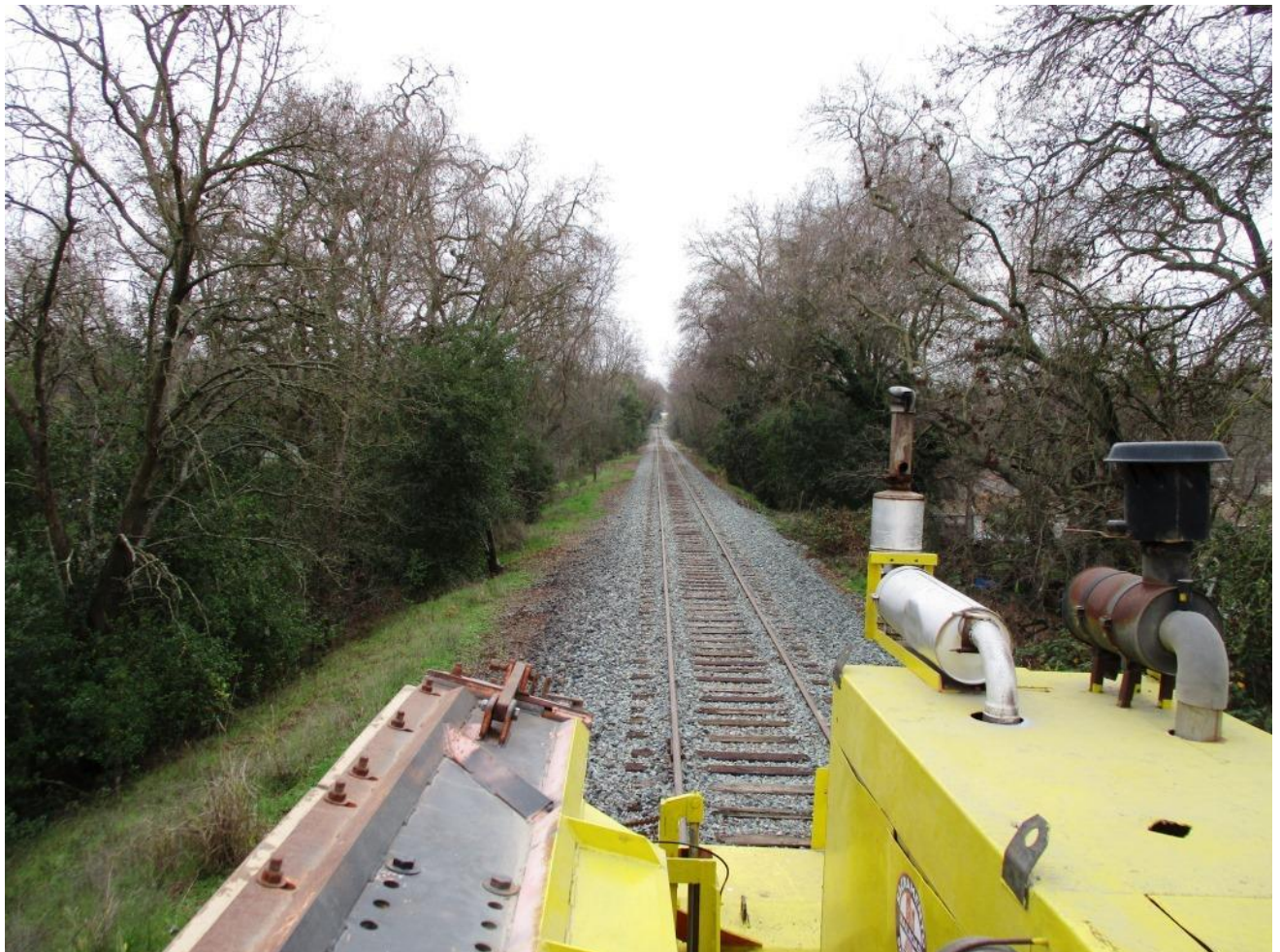
After numerous passes up and down the line using all the regulator's components, Chris C. declares, "The track is DONE!"
