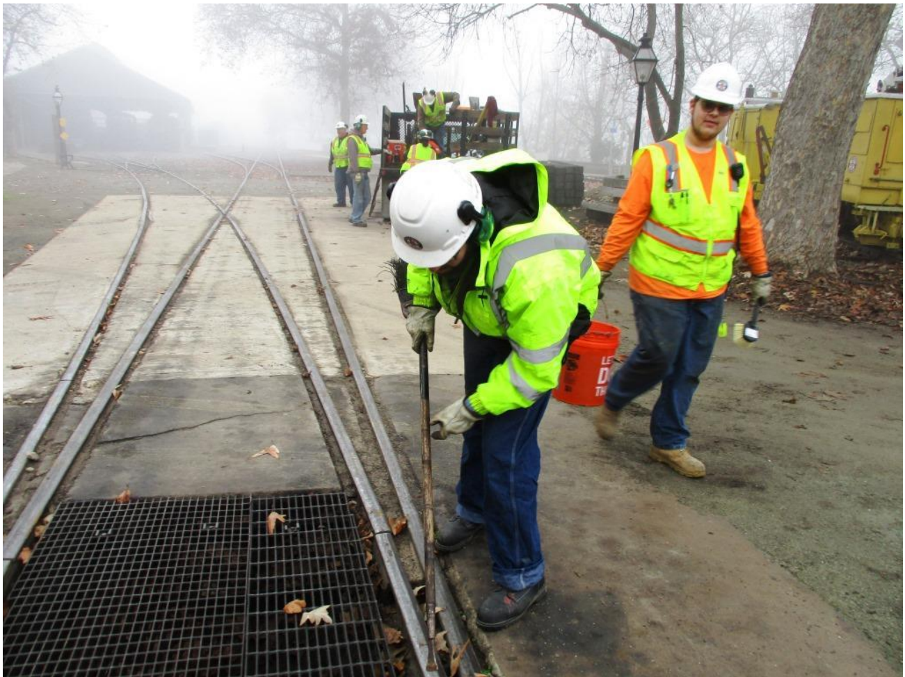
Weston scrapes old dried-up grease and sand from the switch components as Chris H. prepares for his inaugural run with the grease bucket
